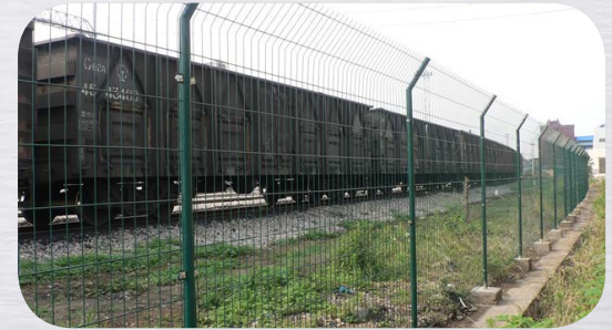
RAILWAY SIDE FENCES
